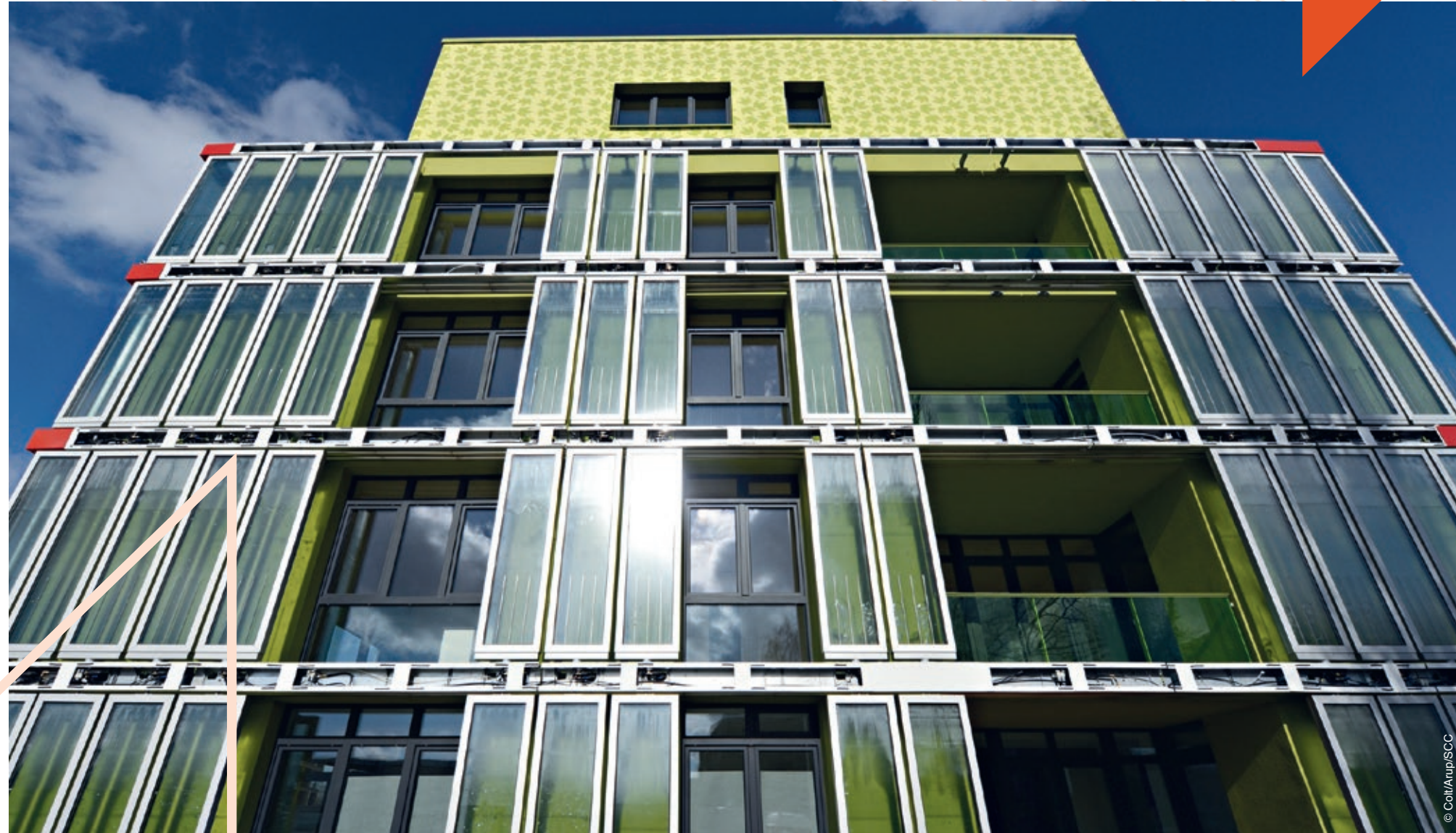
■ The BIQ house piloted the SolarLeaf façade system
