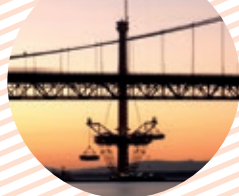
Stonecutters Bridge, Hong Kong with its iconic mono-towers and a cable-stayed span in excess of 1,000m
