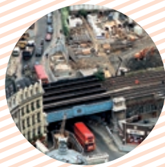
Ludgate Railway Works, London which opened the view of St. Paul's Cathedral by replacing the 1870s railway viaduct with an underground station and restored the railway link between the north and south of the Thames River
