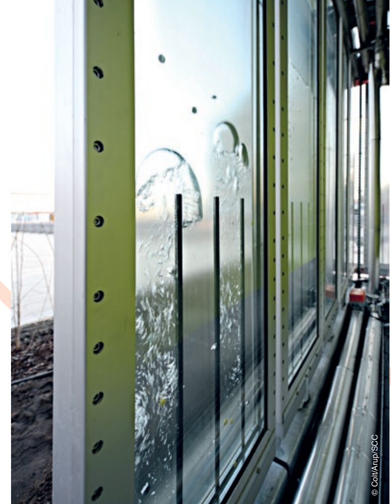
■ A flat-panel glass bioreactor
